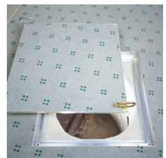
built-in in the office (cleaning shaft), laid out with carpet
